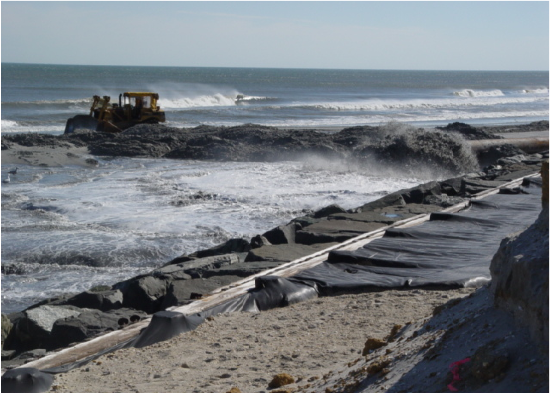
Beach nourishment at Avalon, spring 2008. Photo by Stewart Farrell.
