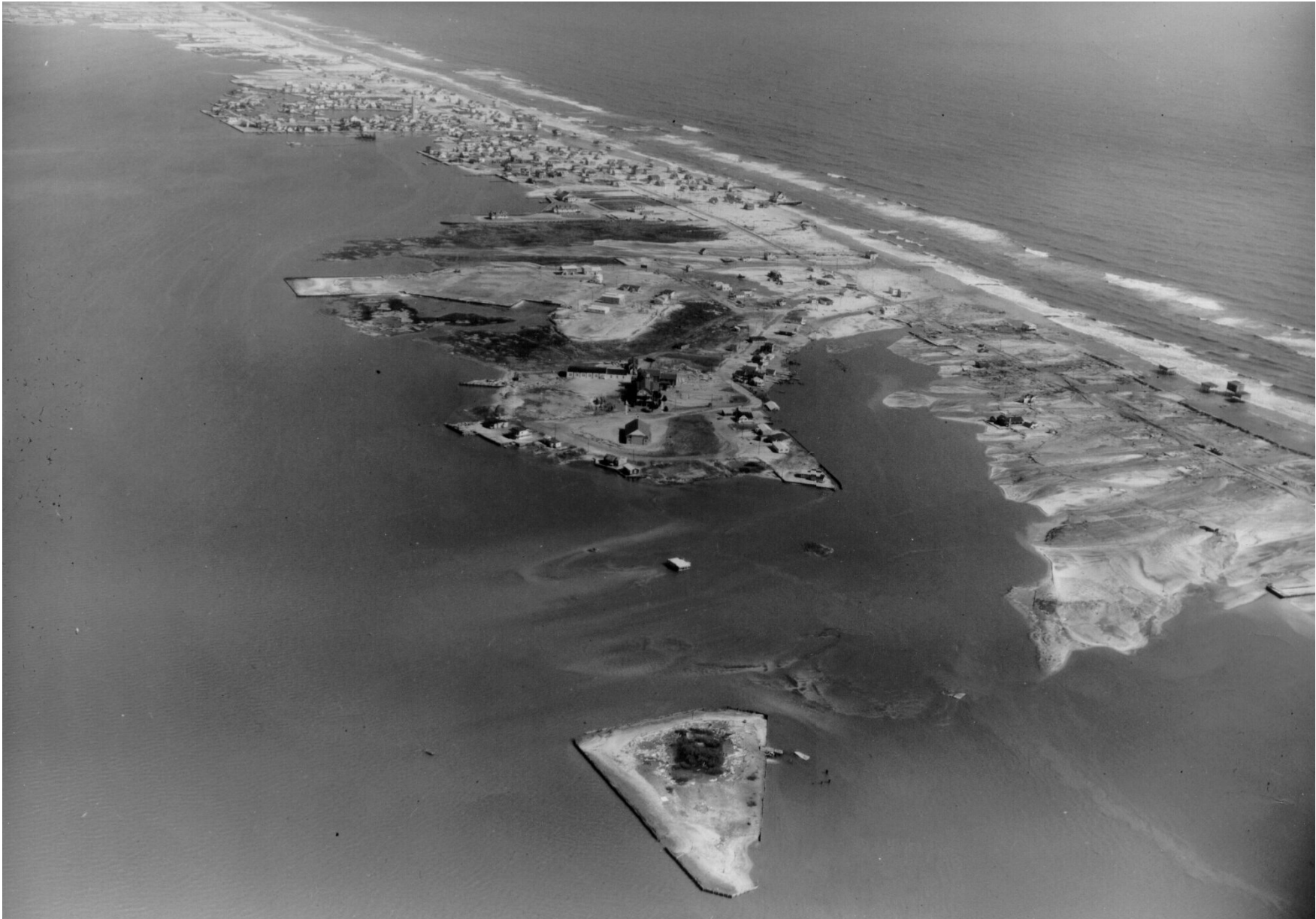
Aftermath of 1962 Ash Wednesday storm, Harvey Cedars Beach. Photo from Harvey Cedars Borough municipal website.
